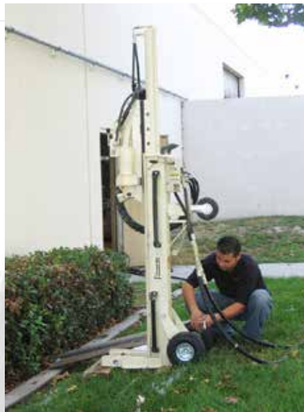
Setting up for 900 linear feet of Macro-Core® borings to 20 feet bgs.
